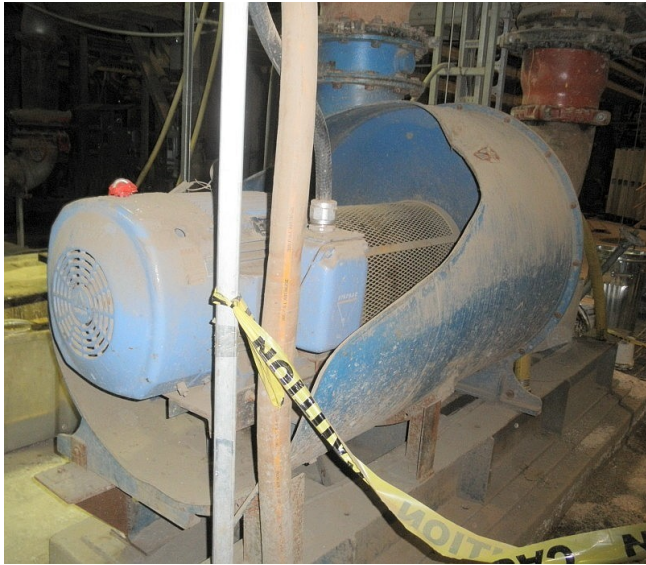
Spencer turbo blower. 75 HP, 3540 RPM, and 12 in. dia. in/out.
