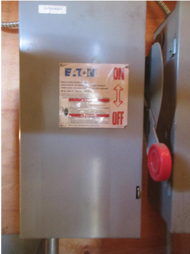
Eaton 60 Amp Fusible Disconnect
